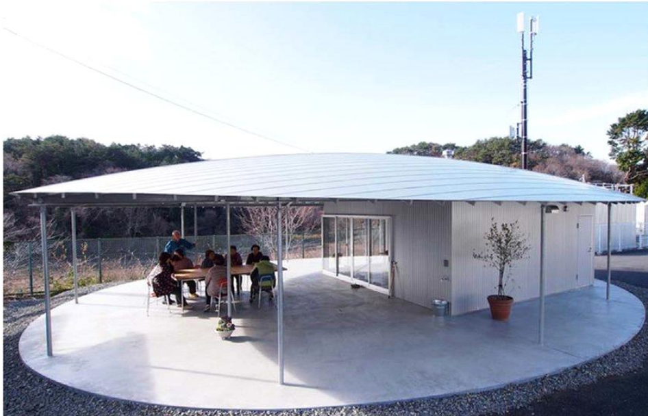
Figure 15 Home for all, Miyato island.
